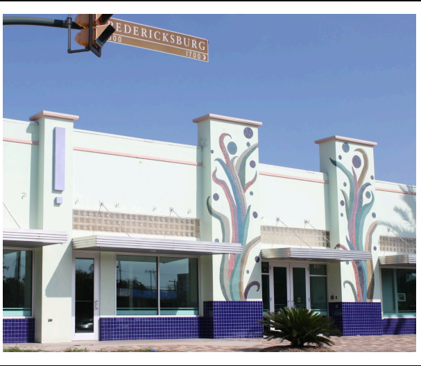
Front of our building
